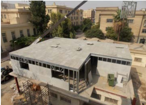
Erection of Ferrocement Slabs and Walls
