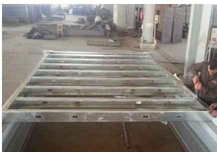
Panel Assembly at Factory
