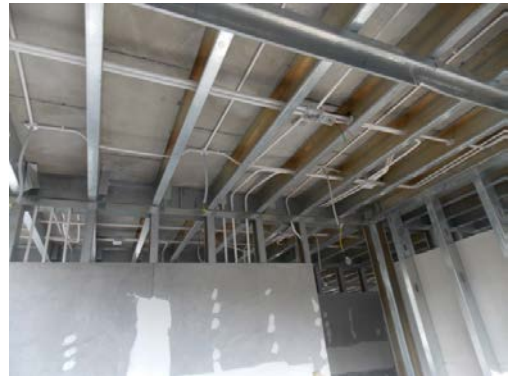
Integration of Services within Walls and Floors during Erection
