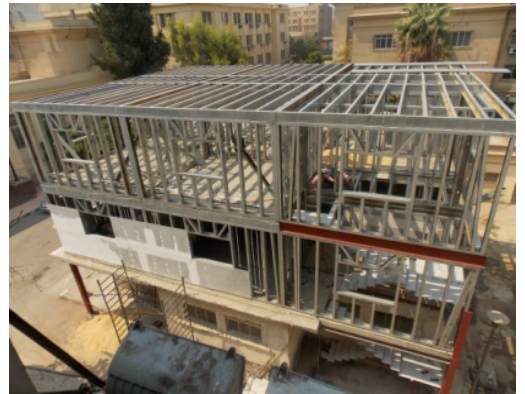
Second Floor Steel Completed
