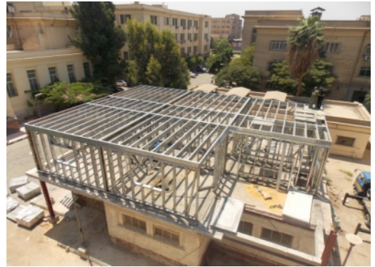
First Floor Steel Erected in THREE DAYS
