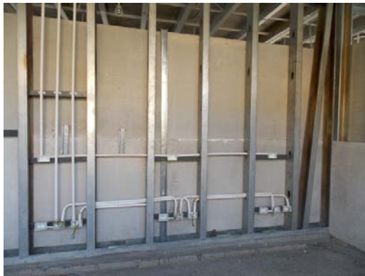
Integration of Services within Walls and Floors during Erection
