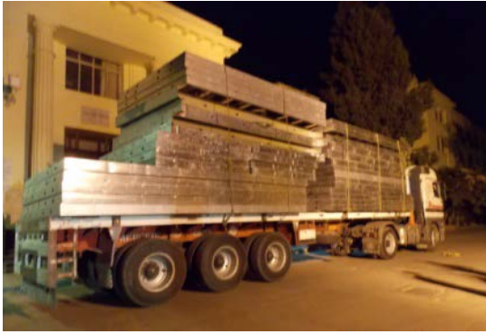
Assembled Panels at site (Entire Floor steel on ONE Truck)
